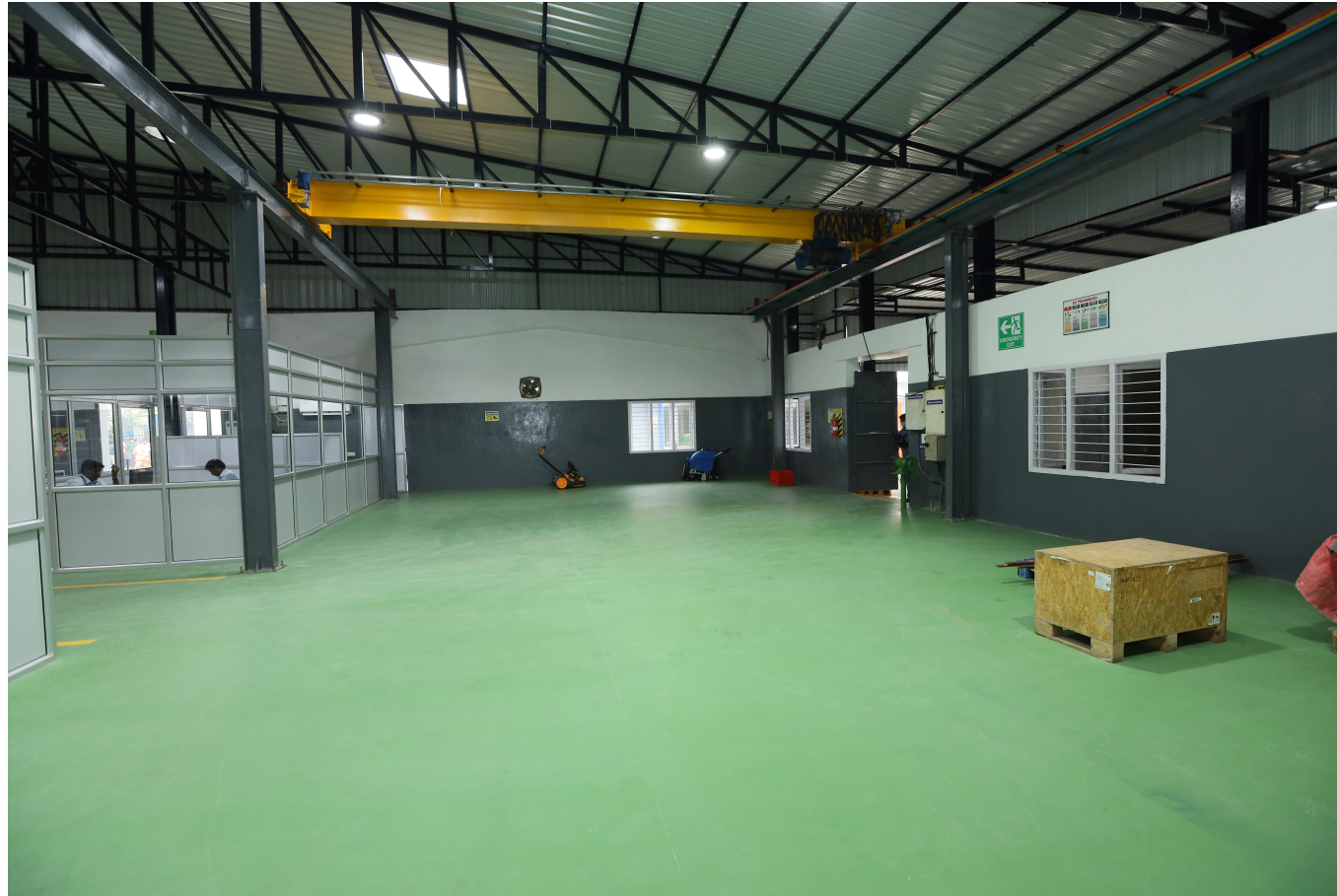
EOT equipped space with performance flooring to handle heavy fabrication needs
